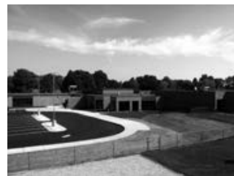
Aerial view of new construction
