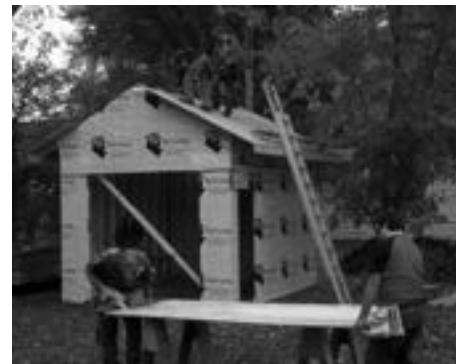
Construction Technology Shed
